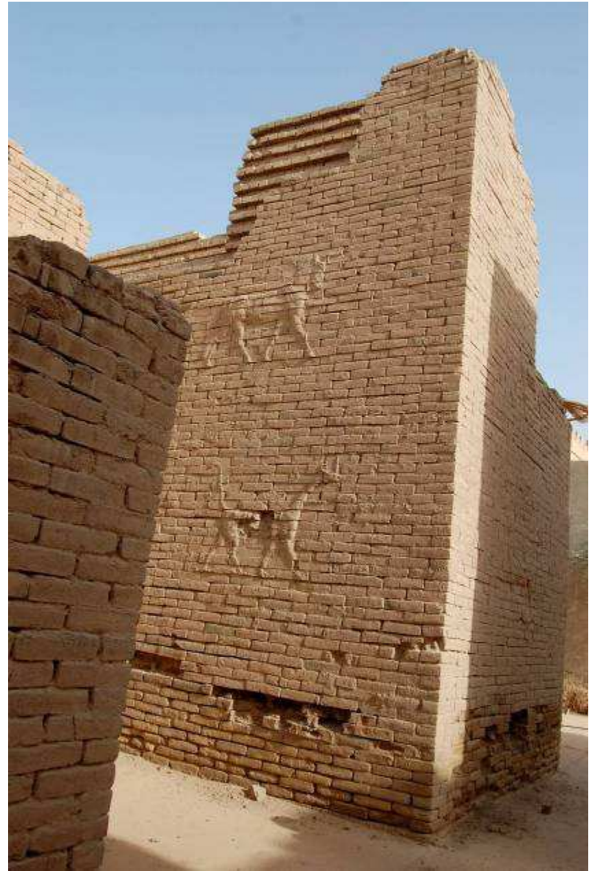
Damage from rising damp, 21 June 09 (Russell photo 229)
