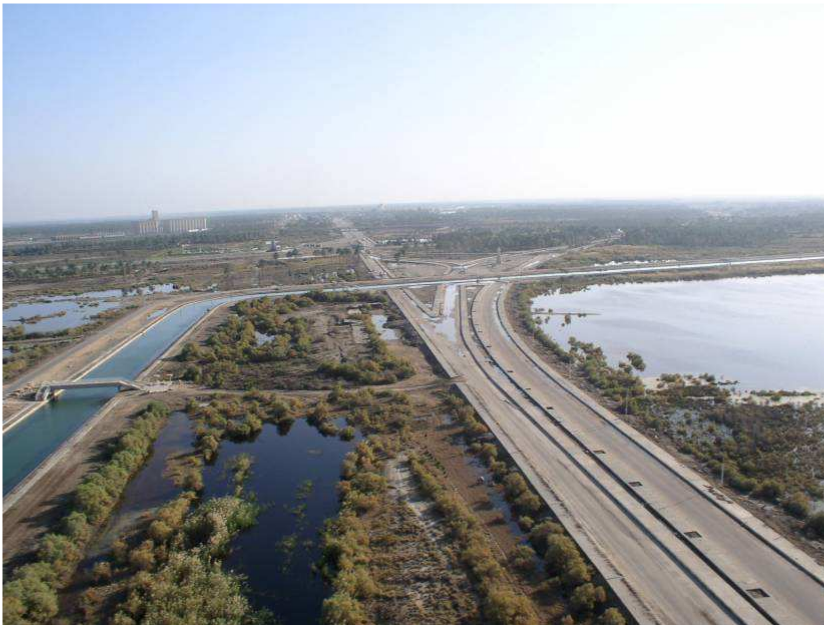
"Al-Hawliyah moat or canal. It surrounds the city of Babylon on the east and partially on the north and south. Its length is 4.5 km and its width is 15 m. The trench is lined on the bottom and sides with cement. This trench is crossed from the north by the main street that links the city of Babylon with the outer perimeter" (Iraqi final report p. 3 and fig. 3).
