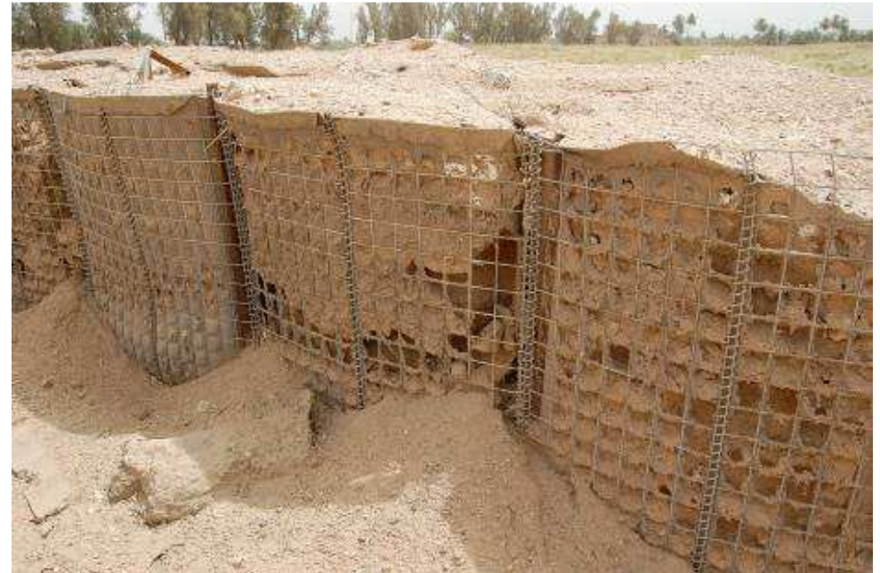
Merkes, Landing Zone 3, deteriorating HESCO containers, July 2008, Russell photo 196 (photo © John Russell)
