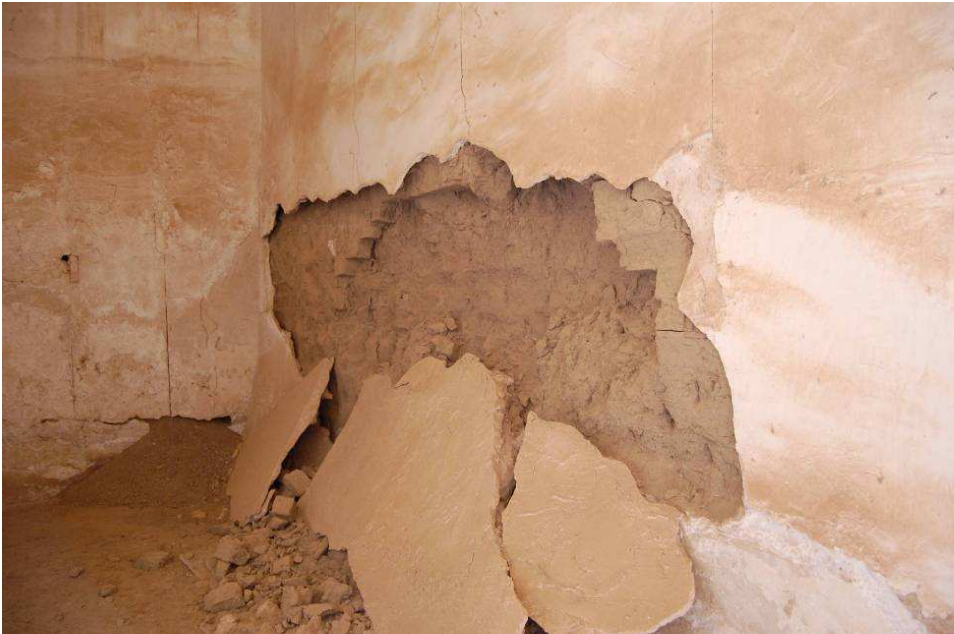
The plaster did not bond with the mud bricks, and is so heavy that in several places it caused large areas of the original brick to shear off and collapse, leaving walls large cavities in their surface (Russell photo 99, 21 June 09, © John Russell)
